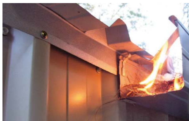
Embers ignite dry leaf litter in roof gutters
